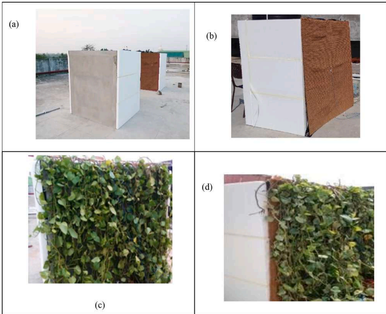
Fig. 3. Photographs of the experimental set-up with four types of insulation skins: (a) Dry coir mat along with bare reference cubicle (b) Wet coir mat (c) Green facade (d) Coir mat with the green facade.
